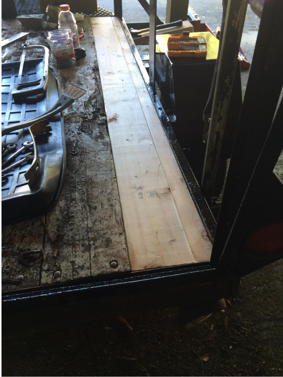
10 - a few floor boards replaced..
