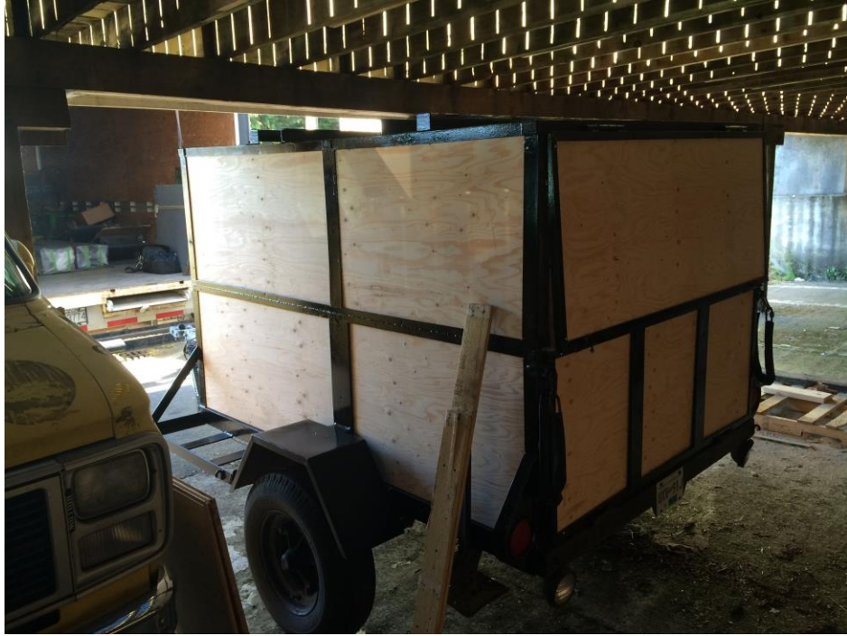
13 - Dry fitting the new walls
